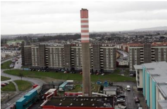
Original Boiler House in Ballymun, Dublin.
