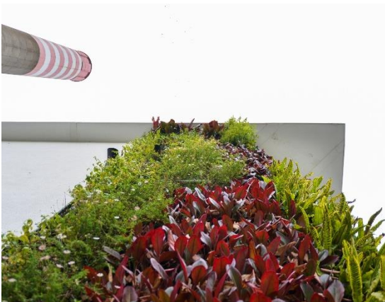
The living wall that also contributes to the insulation of the RDC
