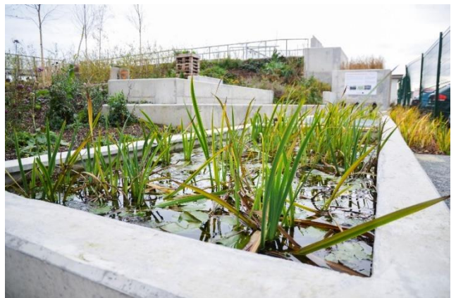
Natural filtration system from the onsite reed bed
