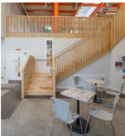
Staircase made from Irish Fir
